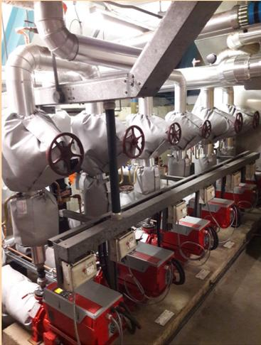
New low temperature hot water pumps with inverters and bespoke insulation jackets have been installed as part of the £1.1 million energy saving upgrade
